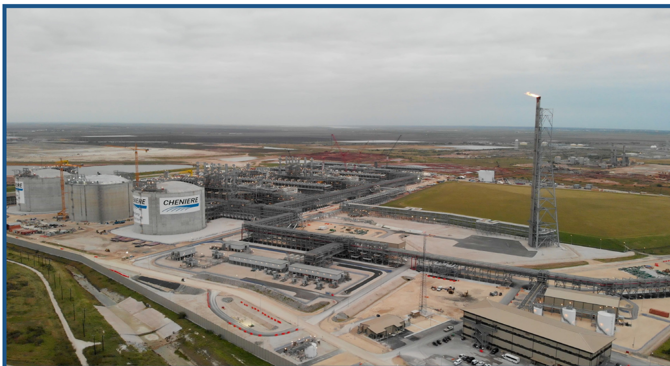
Cheniere LNG facility in Corpus Christi, TX. © Max Anderson of V&M Productions
